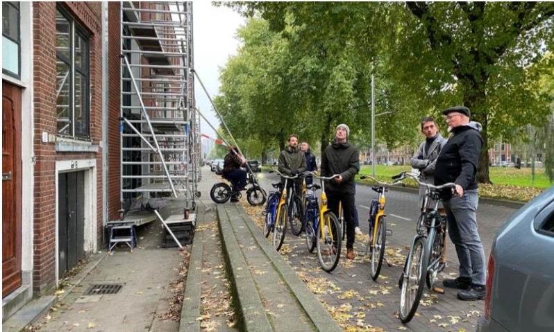
Expedition by the working group in Bloemhof, Rotterdam-Zuid. The houses have subsided compared to the street which used to be at the same level.
