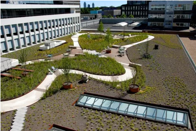
Multifunctional roof with a polder function (water control) in Amsterdam's Zuidas business district.
